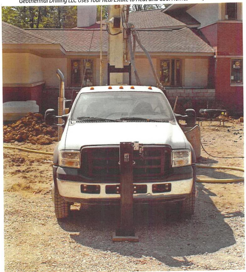
ave. Brennan is in a unique business - capturing the earth's energy for customers. With his company Geothermal Drilling LLC, his crews roll up to a residential home with a drill and a mini ex to install an underground loop system (a series of pipes carrying water and antifreeze) that capitalizes on the constant temperature of the earth to heat and cool homes.
